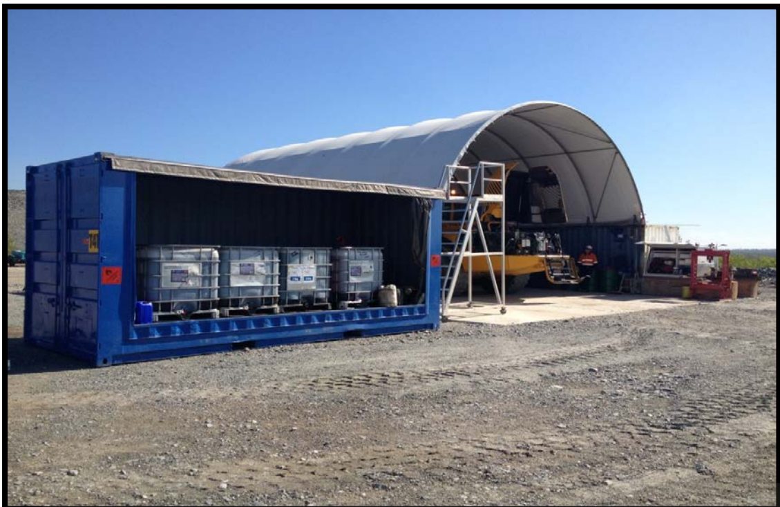
Typical Shaw site workshop and self-bunded waste oil facility. Ranger mine site
